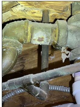
Rusted drain line piping. No leaks observed at the main drain line. The water was off at the time of inspection and no drains were tested for leaks. Replace as needed. (Red)
