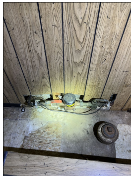
Rusted drain line piping. No leaks observed at the main drain line. The water was off at the time of inspection and no drains were tested for leaks. Replace as needed. (Red)
